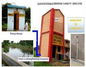
MINI WATER SUPPLY FACILITY WITH SOURCE STRENGTHENING MEASURES
